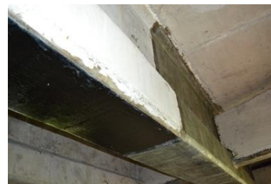
(b) Strengthened girder using GFRP sheet
