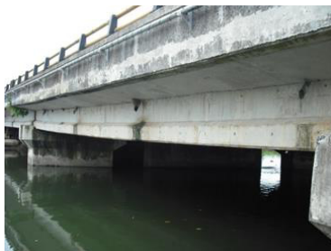
(a) Concrete girder bridge
