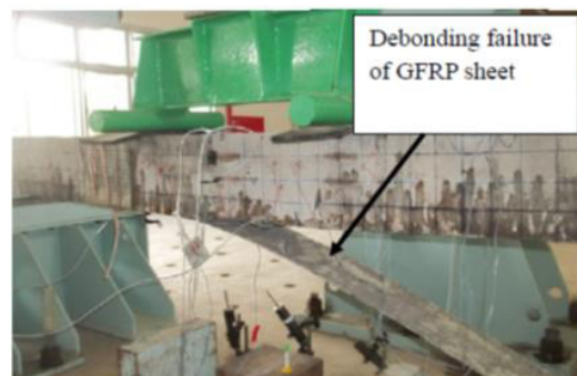
Fig.8. Debonding failure of GFRP sheet.
